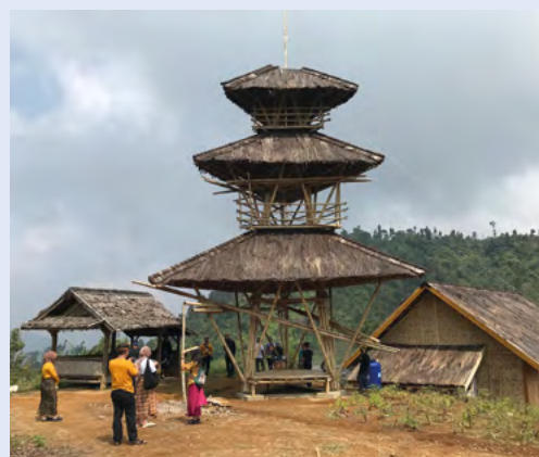
A bamboo local telecoms tower for rural Internet access in Ciptagelar, Indonesia
